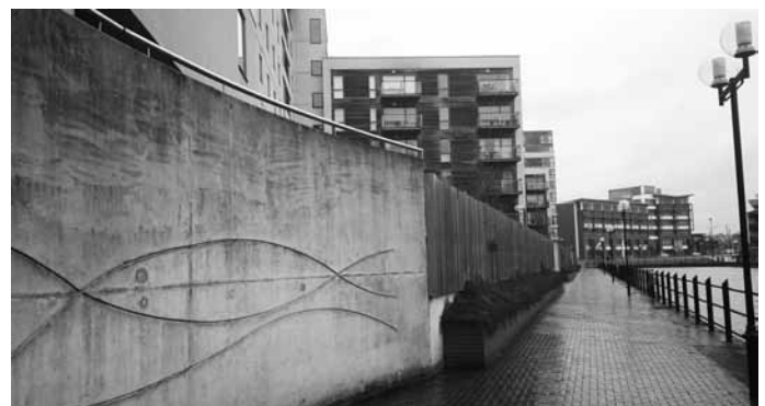
5. Some recent apartments have been designed in an insular or gated form which hasn't always resulted in much pedestrian vitality in their contexts.
