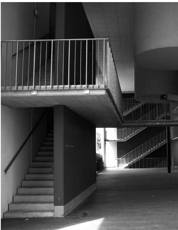
45. We will resist designs that result in public areas of a development which result in blind corners.
